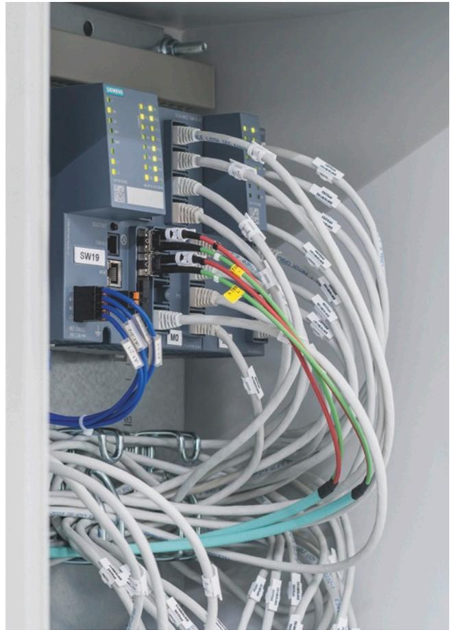
A total of 95 Scalance X switches form the interfaces of a network structure made up of multiple subnets, e.g., consisting of Scalance XM416-4C ....
