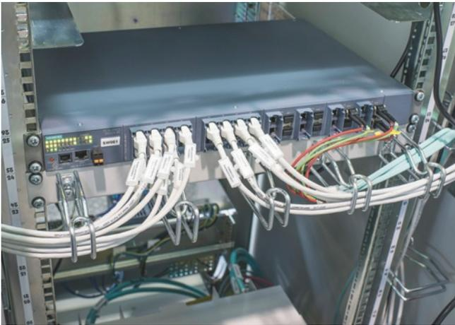
The managed switches SCALANCE XR528-6M with device network management from Siemens are connected with a 1 Gbit line.
