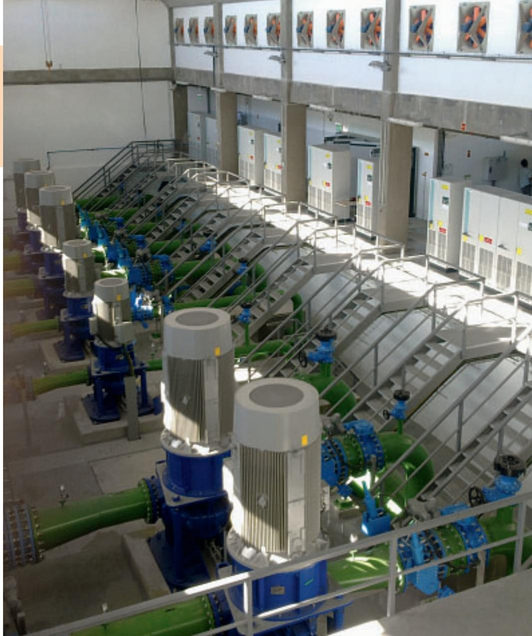
rate can be set much more precisely and with shorter response times than with throttles or valves. In case of fluctuations in demand, the pump can also adapt the output to the current demand much more quickly and exactly. Not least, the soft starting and stopping relieves the mechanics of the drivetrain, thus increasing its service life. Pressure waves that cause stress or even damage do not occur in the pipe systems here.
