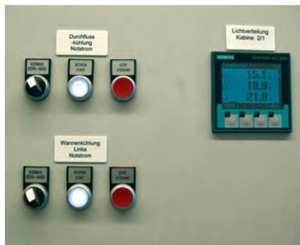
▲ Saint-Gobain Oberland’s plants already had measuring points such as the 7KM PAC 3200 power monitoring device which could be easily incorporated in Simatic B.Data.
