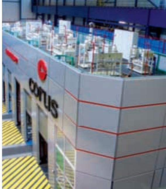
New PLTCM linked to an existing pickling line at Corus, Netherlands
