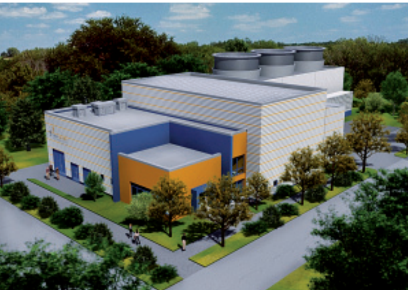
Outside view of the Unterhaching geothermal power plant (computer animation)
