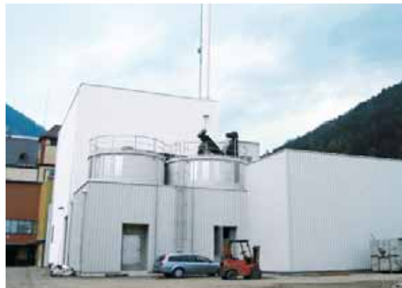
Reject Power plant in Hirschwang, Austria, for the on-site conversion of 10,000 metric tonnes of waste annually into steam and electric power. This plant can supply up to 30 percent of the power required for production.
