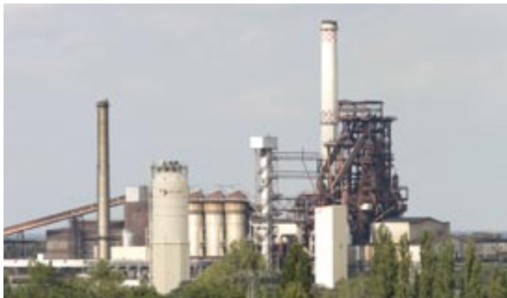
Blast furnace 5A, ArcelorMittal, Eisenhüttenstadt, Germany
