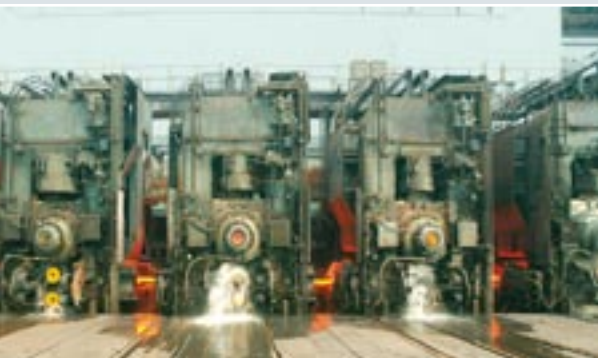
5-Stand finishing mill (Existing ISP plant)
