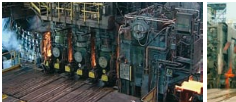
Continuous caster with integrated 3-stand high-reduction mill (Existing ISP plant)
