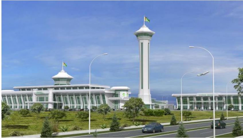
The Turkmenbashi Airport (KRW) in Turkmenistan (Photo: Polimeks Construction Company)
